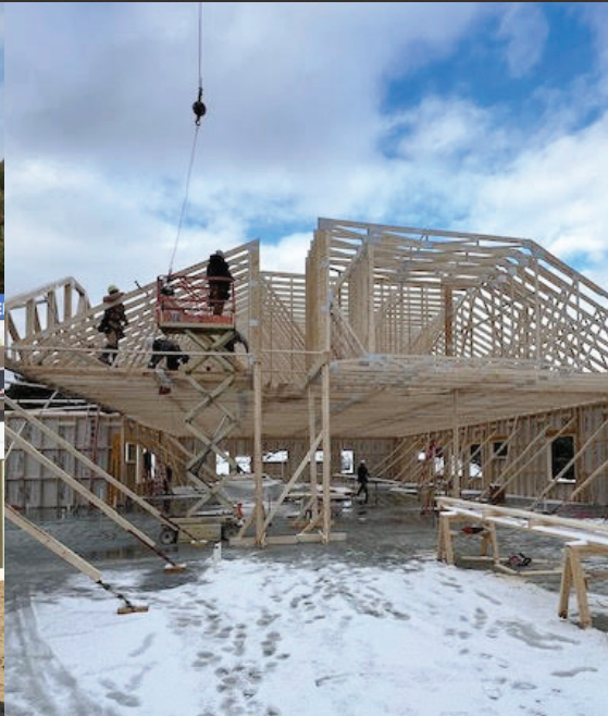
By the end of December, trusses for the roof of the 10,000-square-foot building were in place.
